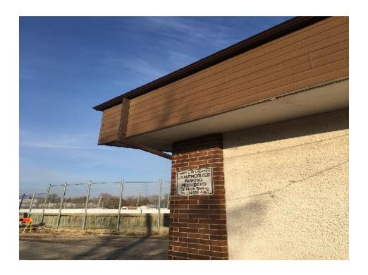
Figure 6: Match existing CanExcel Siding.
