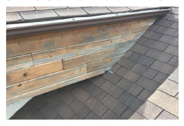
Figure 9: New siding throughout including all counter-flashings and step flashings.
