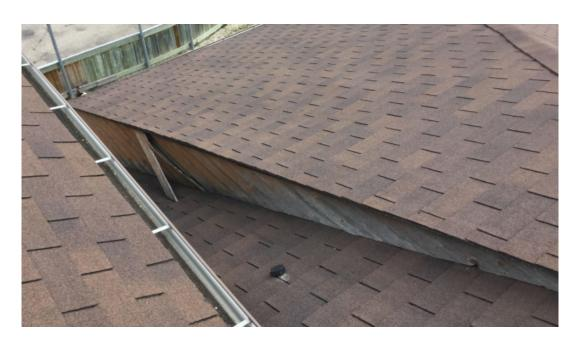
Figure 7: New siding at gable ends adjacent to shingle elevations. Base flashings should be provided for b/w siding & shingles.
